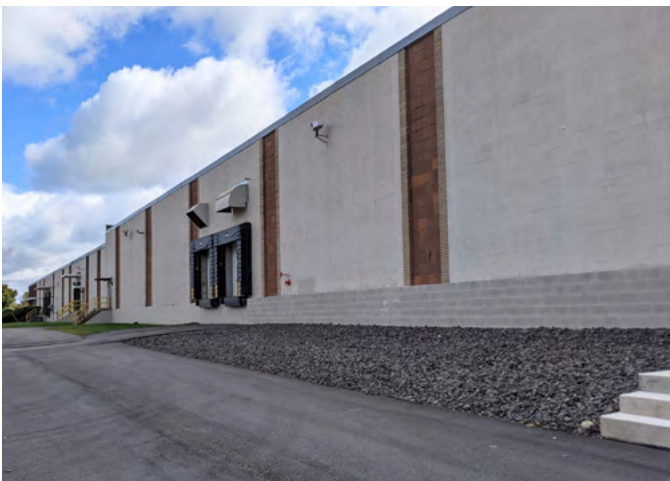
NPC Global Newly Paved Truck Court Area
